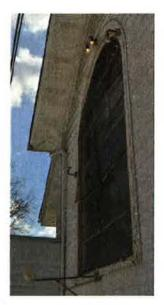
glass replaced and soldered, panels waterproofed two sides, Lexan panel installed, and new steel bars attached." 701sca, 689sca.
